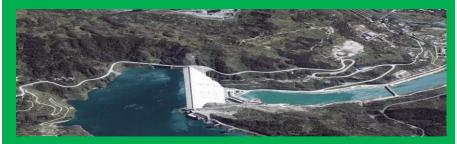
In order to prevent the uncontrolled rapid release of water from the reservoir of a storage dam during a strong earthquake, Large storage dams are generally considered safe if they can survive an event with a return period of 10,000 years, i.e. having a one percent chance of being exceeded in 100 years.
